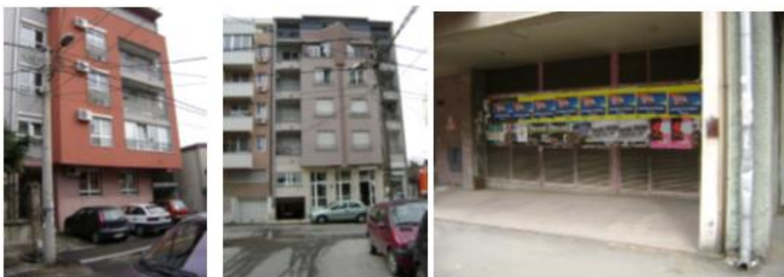
Figure 18,19 and 20. "spiderman" nets and multi-story building with a sub-station on the ground floor
